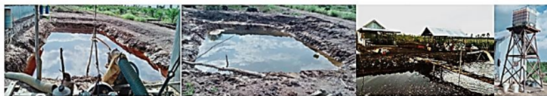
Kolam penampung; Kolam treatment ; pompa air; tandon
