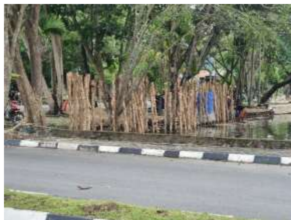
Figure 4. Gelam wood as lateral reinforcement
