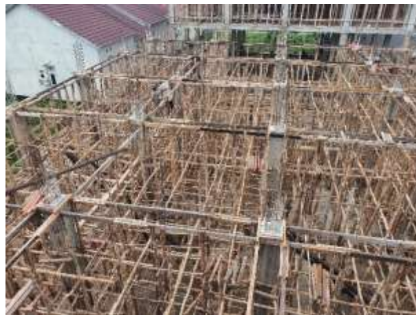
Figure 5. Use of gelam wood as a scaffolding
