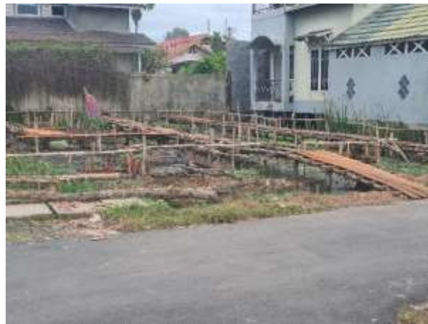
Figure 3. Gelam wood foundation for residential houses
