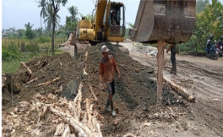
Fig. 6 Gelam wood foundation for road construction [25]
