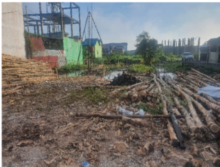
Fig. 2 Gelam wood piles on the construction site
