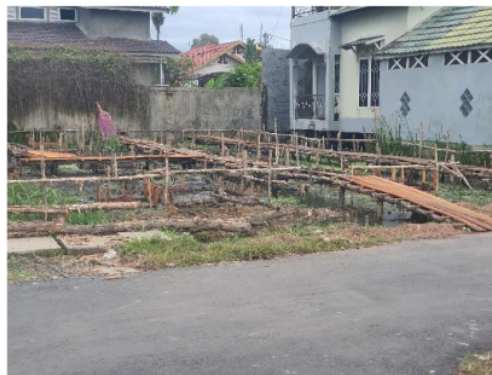
Figure 3. Gelam wood foundation for residential houses
