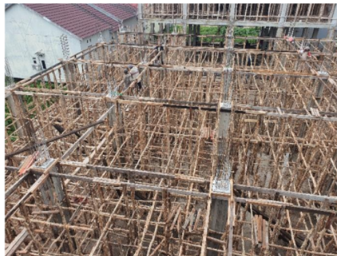
Figure 5. Use of gelam wood as a scaffolding
