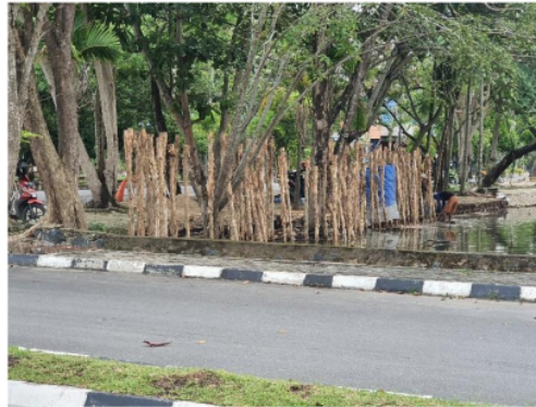
Figure 4. Gelam wood as lateral reinforcement
