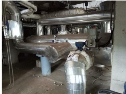
Gambar 1. Gland Steam Condensor
