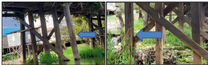
Figure 5. Tampa Bridge Condition during Investigation
