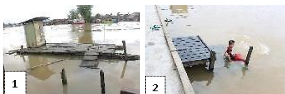
Figure 1. Batang lanting with a floating bamboo construction (1) and batang panggung with an ironwood construction (2)
