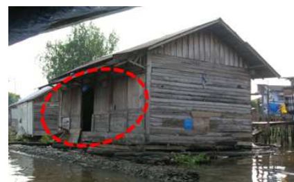
Figure 7a. Building orientation in the present condition. In the past, the lanting house function as a shop, but now is changing become a house for living only
