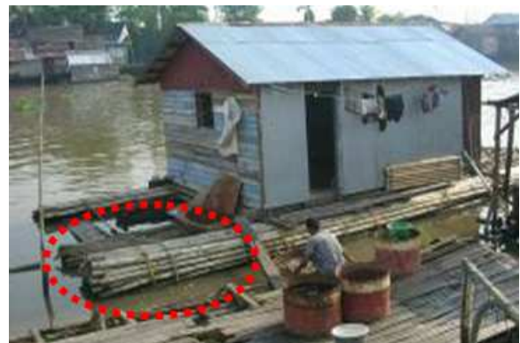
Figure 10. Foundation Construction in present condition is using bamboo
