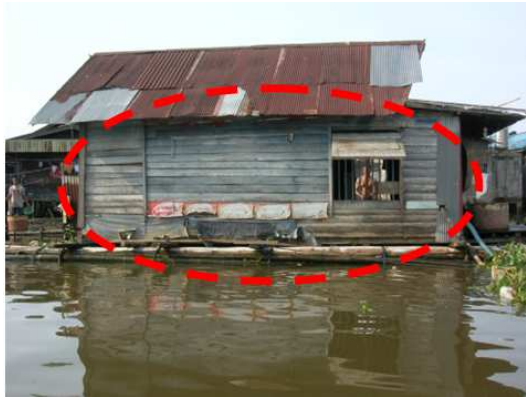
Figure 7b. Building orientation in the present condition. lanting house orientation was changed towards the land. Shop function is non-existence.
