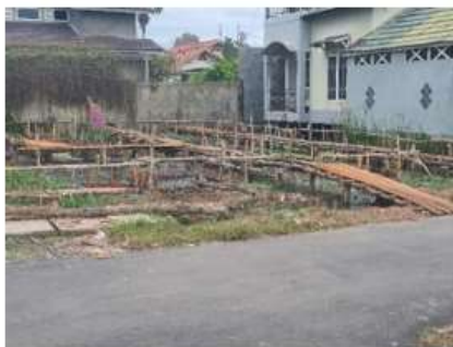
Figure 5. Gelam wood foundation for houses
