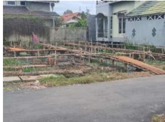
Figure 2. Gelam wood foundation for residential houses
