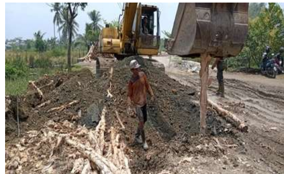
Figure 3. Gelam wood foundation for road construction [24]
