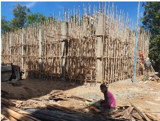
Fig. 9 Gelam wood as a scaffolding
