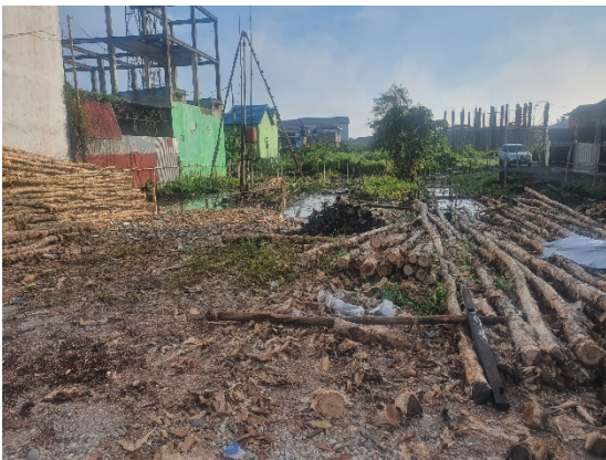
Fig. 2 Gelam wood piles on the construction site
