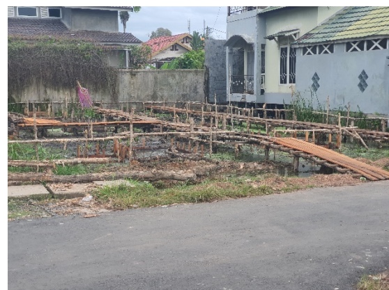
Fig. 5 Gelam wood foundation for houses
