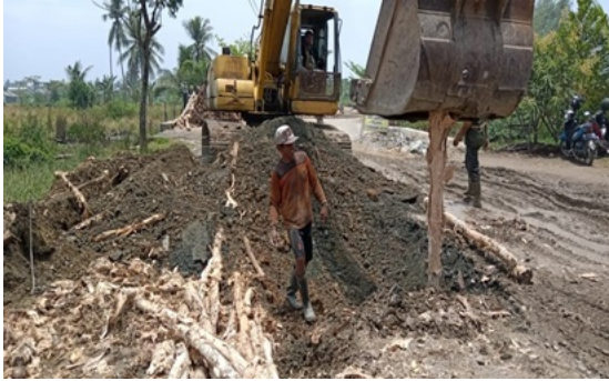
Fig. 6 Gelam wood foundation for road construction [25]
