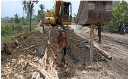
Fig. 6 Gelam wood foundation for road construction [25]
