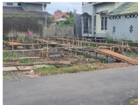
Fig. 5 Gelam wood foundation for houses
