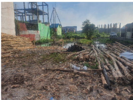
Fig. 2 Gelam wood piles on the construction site
