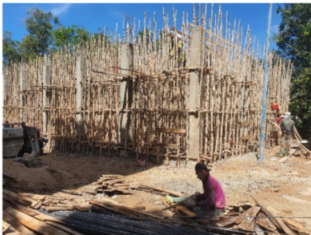
Fig. 9 Gelam wood as a scaffolding
