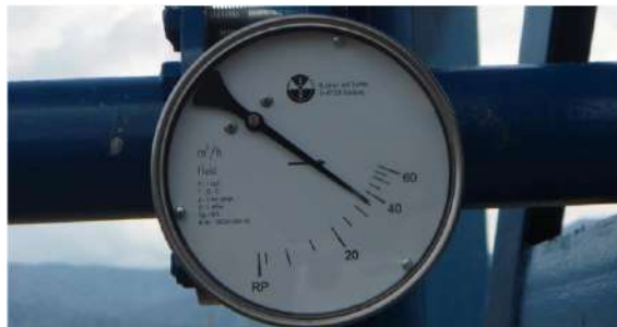
Gambar 6. Flow meter SPAM IKK, Kab. Majene, Sulawesi Barat (Sumber : Prasarana dan Sarana Air Minum, 2015)
