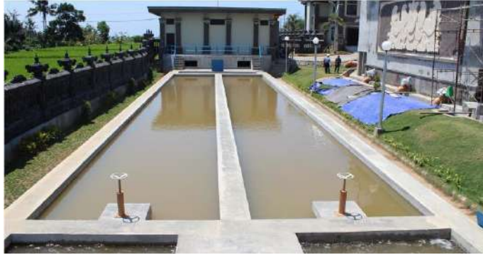
Gambar 7. Bak prasedimentasi SPAM Regional Kab. Gianyar, Bali (Sumber : Prasarana dan Sarana Air Minum, 2015)
