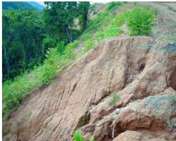
Figure 3. Cutting Slope as Triggering Factor for Rotational Landslide
