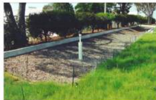
Gambar 6-15 Detail Infiltration Trench
