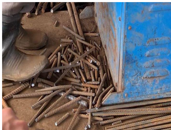
Fig. 1 Remaining Pieces of Steel Reinforcing
