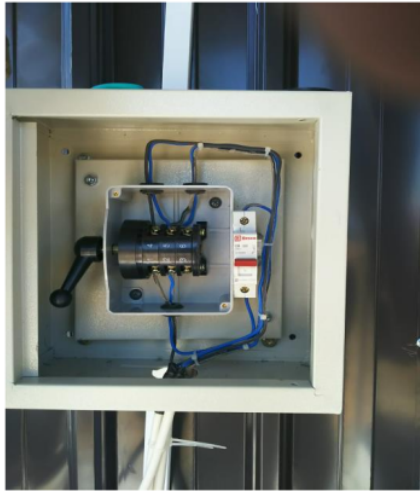
Gambar 8 Instalasi Box Panel
