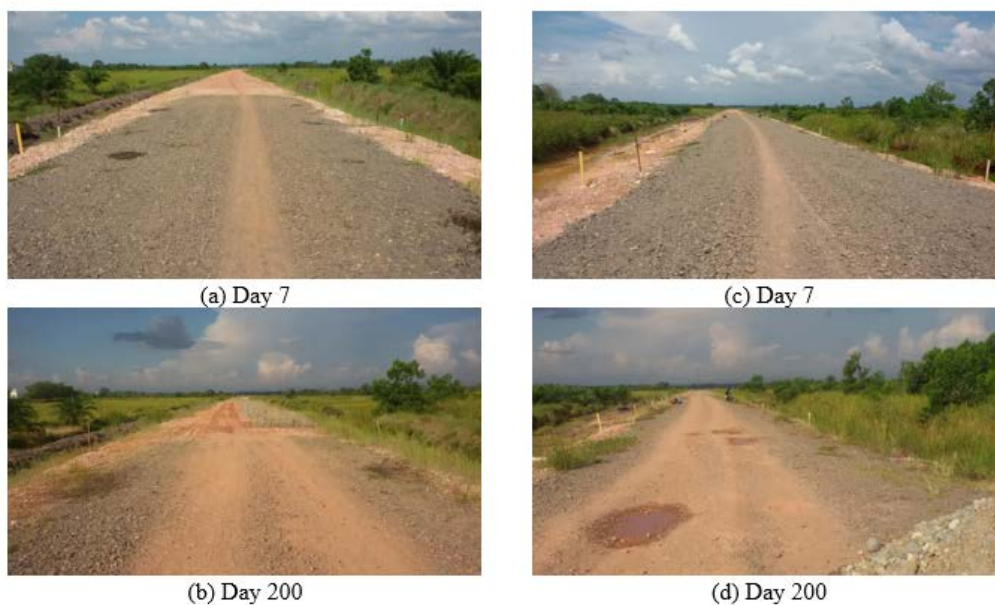
Fig.7 Photo Visual Field Observation (a, b) Embankment 1, and (c, d) Embankment 2
