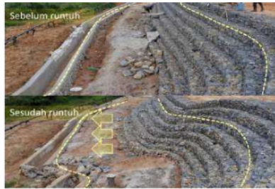
Figure 1.1 Deformation of Shapes in Gabion Construction.
