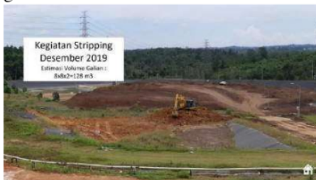
Figure 4. 9 Excavation Activities at the Foot of the Slope.
