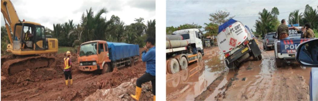
Figure 1: Lateritic soil as a subgrade road condition
