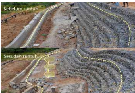
Figure 1.1 Deformation of Shapes in Gabion Construction.
