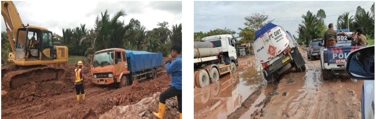
Figure 1: Lateritic soil as a subgrade road condition
