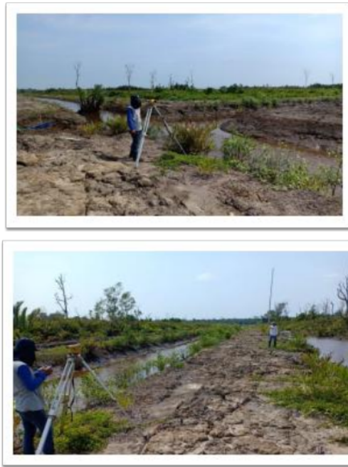
Figure 2 Measurement of the existing embankment elevation in primary channel IV
