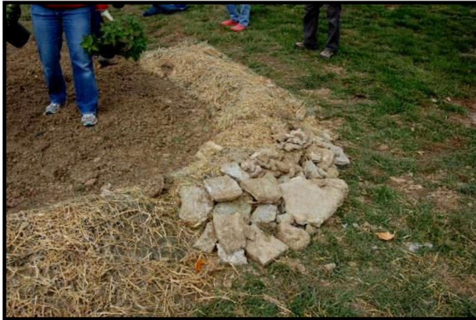
Gambar 7. Membangun Daerah Penahan Limpasan Air ( http://www2.ca.uky.edu/gogreen/images/green/boone_berm.JPG ).
