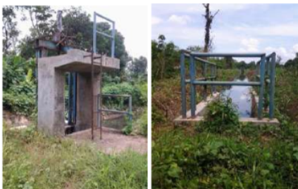
Fig. 8 Irrigation channel in Polder Liang
