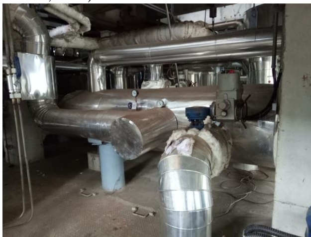
Gambar 1. Gland Steam Condensor
