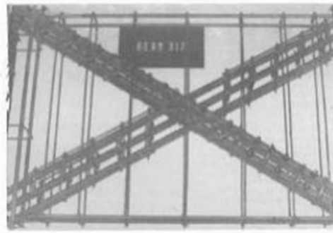
Fig.2. Typical Layout of diagonally Reinforced Coupling Beam [2].
