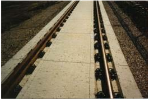
Fig. 3. Example of application of ACC on CRCP in Germany
