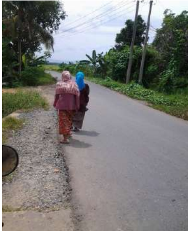
Fig. 7 Dikes as paved road in Liang Polder
