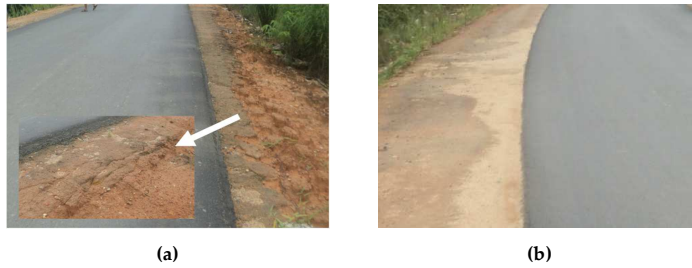
Figure 1. The appearance of soil-cement as a base (a) undergo wetting-drying cycles, and (b) non submerged road
