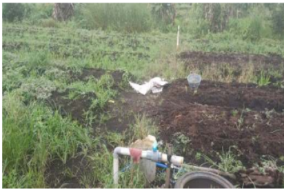
Figure 1 Drilling Well Located on Community-Owned Land Community
