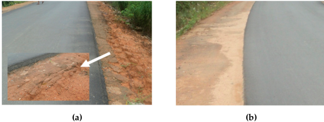
Figure 1. The appearance of soil-cement as a base (a) undergoing wetting–drying cycles, and (b) non-submerged road.
