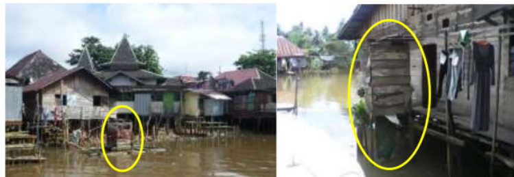
Figure 7. Condition of the toilets on the banks of Kuin River (source: Field Documentation, 2020)
