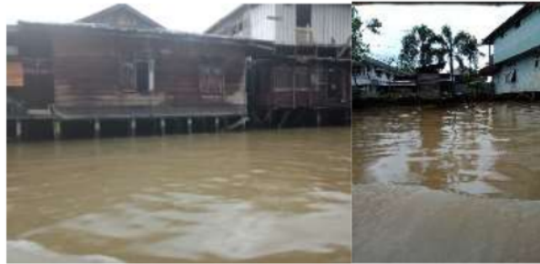
Figure 5. The condition of the houses on the banks of Kuin River (source: Field Documentation, 2019)
